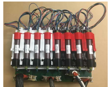
Batteries and Cells tested to RCC 319-14
